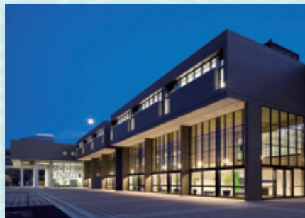
Gate Plaza (Building 1)
